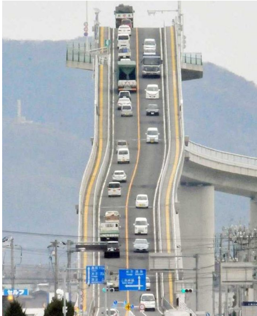
Eshima Ohashi Bridge in Matsue, Japan
